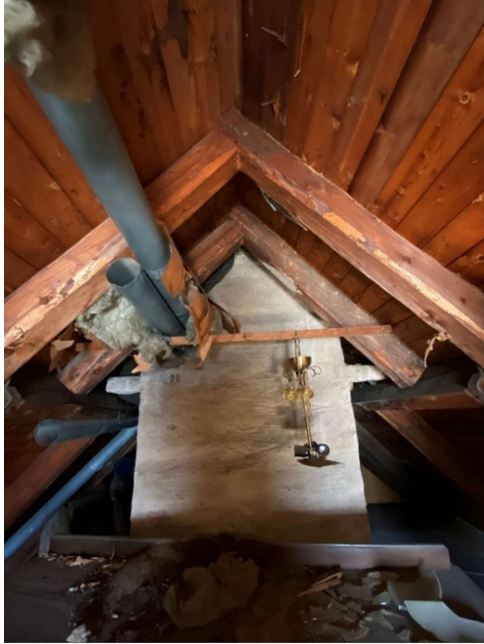
Figur 3-7 – Skorsten under taket
